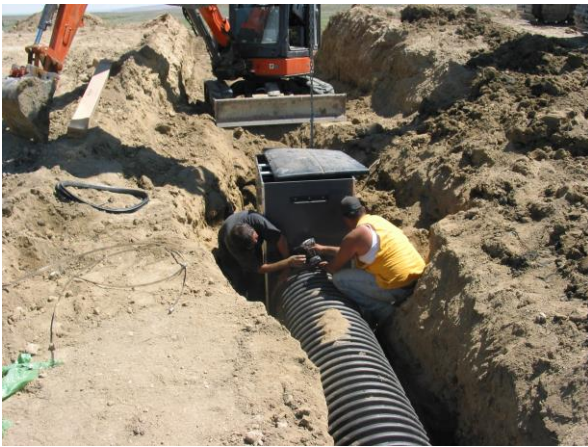
Tribal Construction Company installing water control structures.
