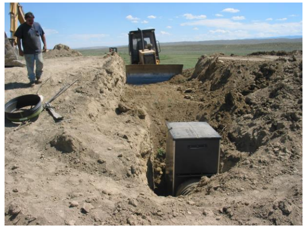
(After) Repaired dike with head-cut correction
