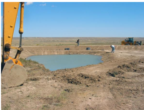
Newly constructed reservoir/junction box to split produced water flows into two different drainages.
