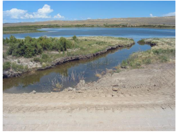
(After) Repaired dike with head-cut correction
